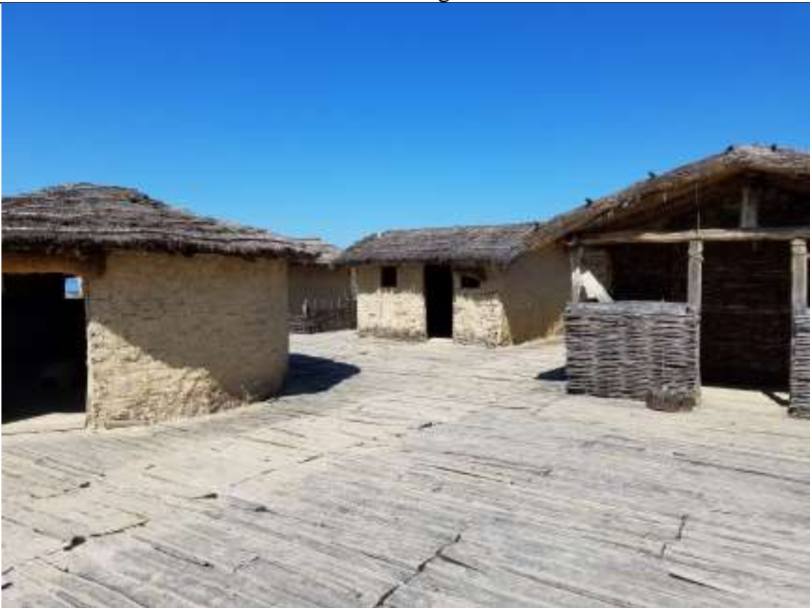
Reconstructed Houses on the piles in the lake
