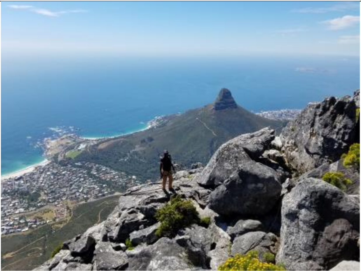
On top of "Table Mountain" workman with no dear working on cables at edge
